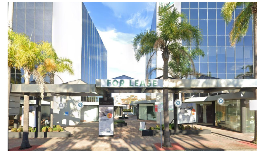
Existing building front entrance
