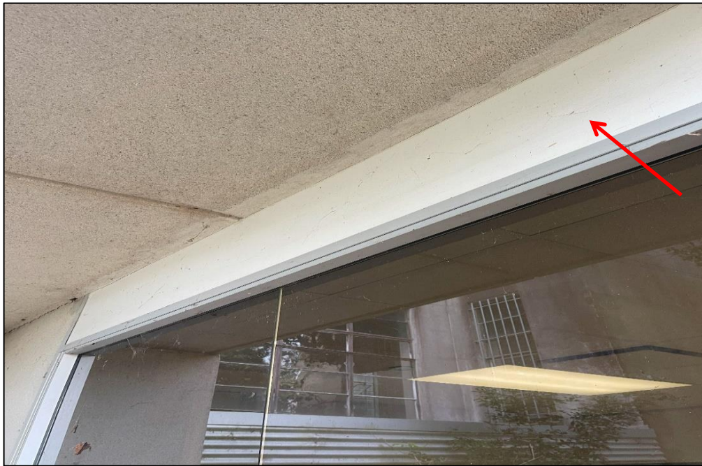
Photograph 4: North Tower, exterior, western end, infill panel, suspected non-asbestos.
