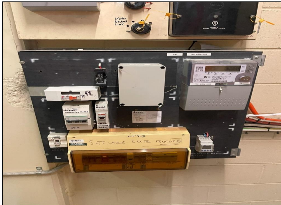
Photograph 30: Basement car park, services room, electric backing board, suspected non-asbestos.
