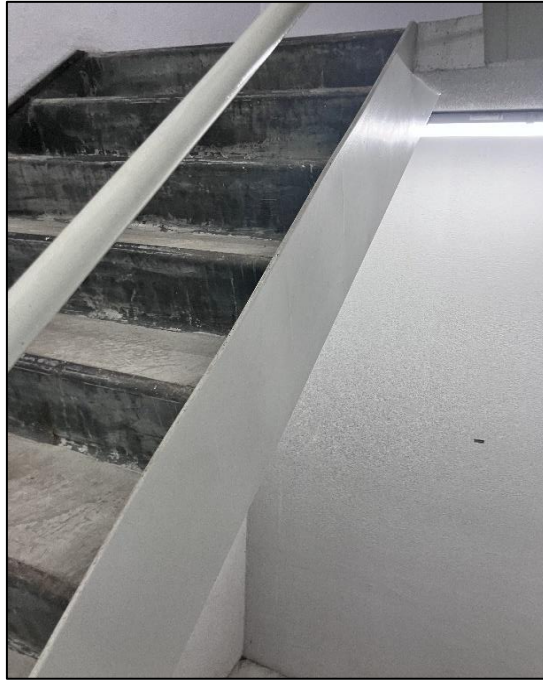
Photograph 55: South Tower, main stairwell, metal facing to stairs, white paint.
