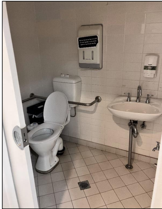
Photograph 41: South Tower, Levels in general, lift foyers, amenities generally, below ceramic floor and wall tiles, substrate, inaccessible.
