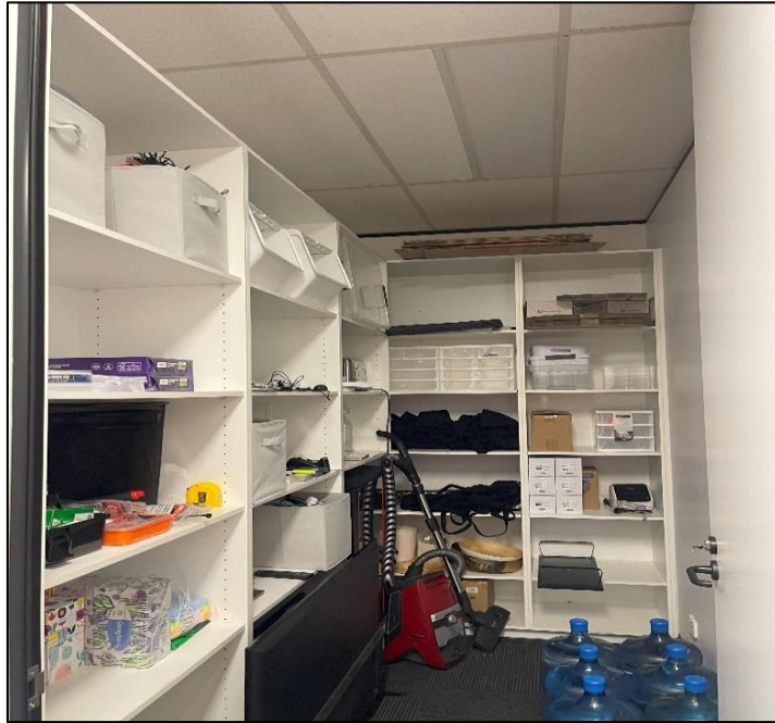
Photograph 15: North Tower, tenanted offices / retail shops, throughout, materials in general, limited access, suspected non-asbestos.
