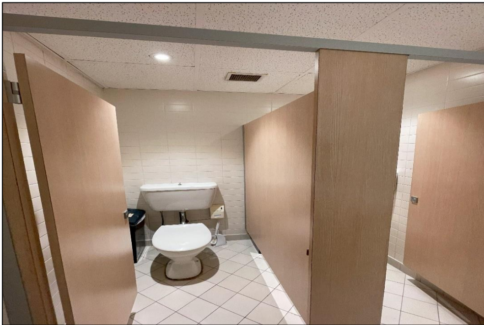
Photograph 10: North Tower, level 4, toilets, below ceramic tiled walls and floors, substrate, inaccessible.
