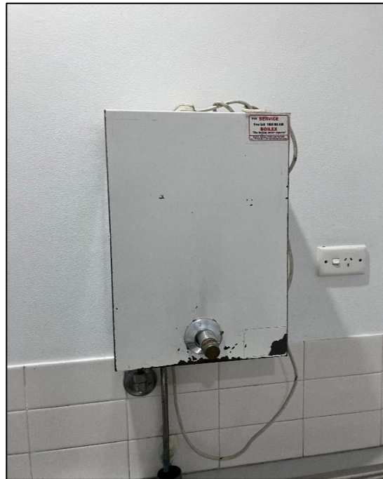
Photograph 52: South Tower, Ground Level, mailroom corridor, boiling water unit, insulation, inaccessible.
