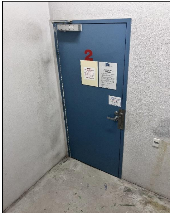
Photograph 54: South Tower, main stairwell, typical doorframe, blue paint.
