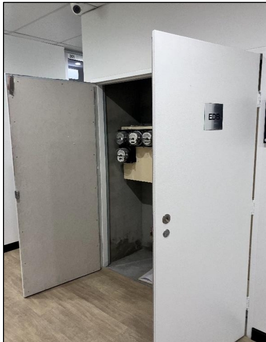
Photograph 36: South Tower, Level 3, lift foyer, EDB cupboard, doors, fibre cement linings, no asbestos detected by analysis.
