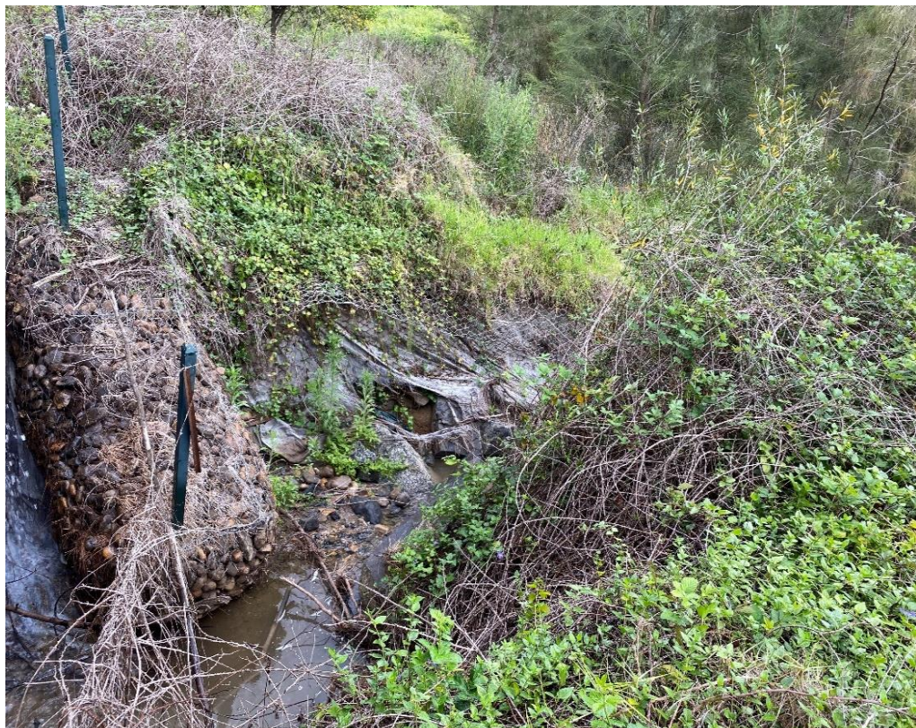
Photo 6: Existing Stormwater Channel adjacent to BH16
