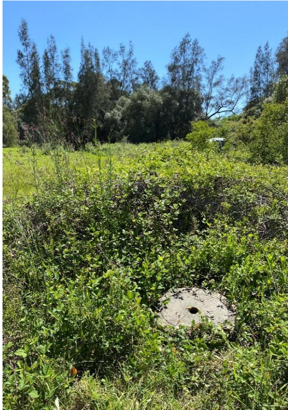
Photo 5: Existing Sewer Mainhole adjacent to Site Boundary Fence
