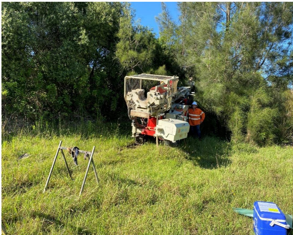
Photo 3: General Site Condition adjacent to BH15 Looking West
