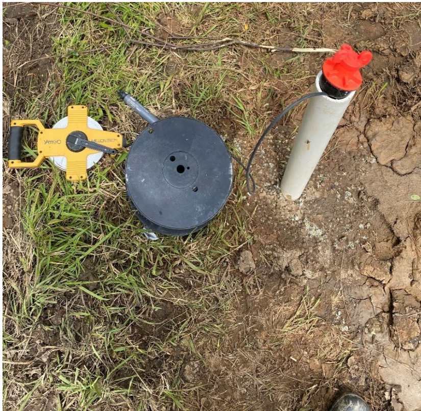
Photo 8: Typical Piezometer Setup with a HOBO
