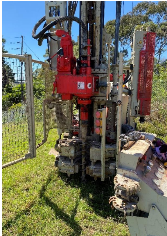
Photo 7: Typical Drill Rig Setup
