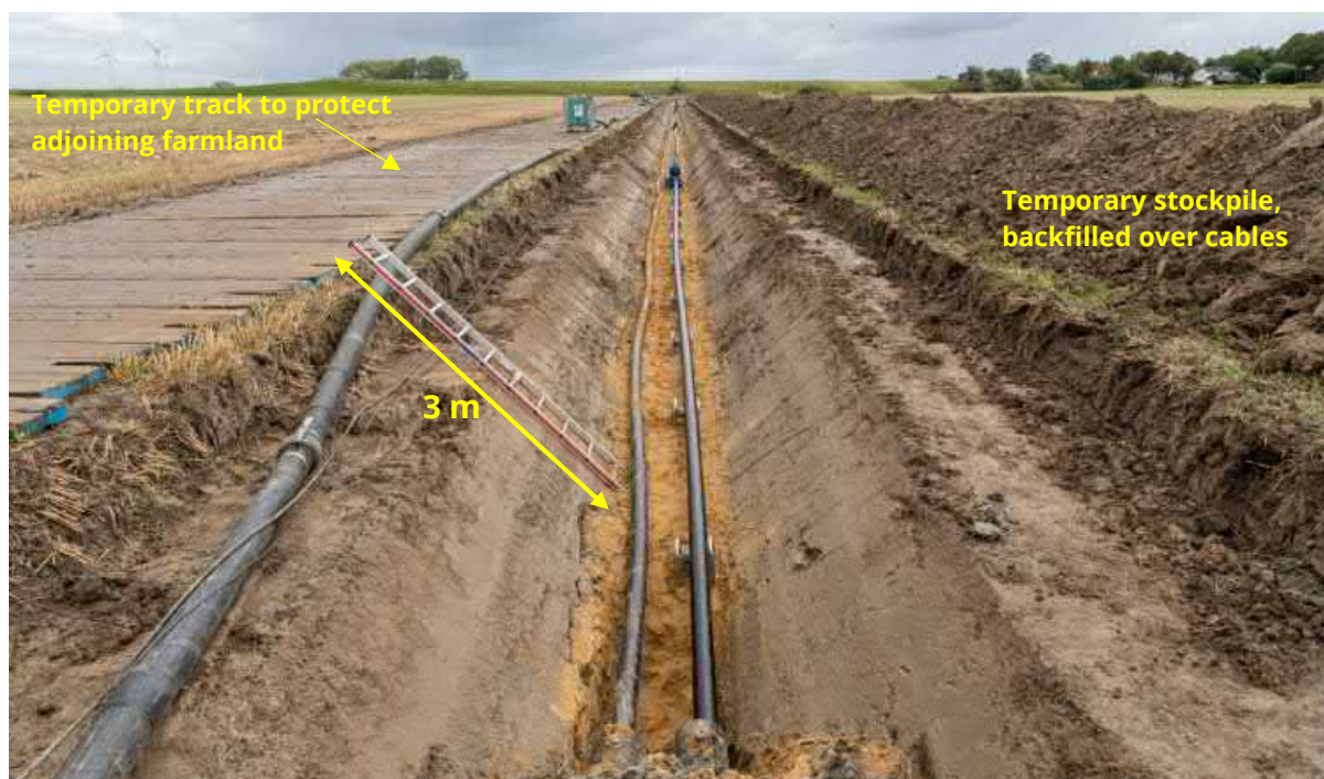
Figure 1. Construction of the 500 km long 525 kV SuedOstLink in Germany using construction corridor of minimum width necessary, as would be required in Australia. The construction corridor appears to be close to the 11.5 m width quoted above with another 3 m on each side for access and stockpiling excavated material, totalling 17.5 m. Source: TenneT
