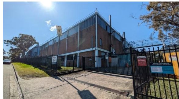
Figure 2.18 Southwestern corner of the warehouse building at 82 Hughes Avenue.
