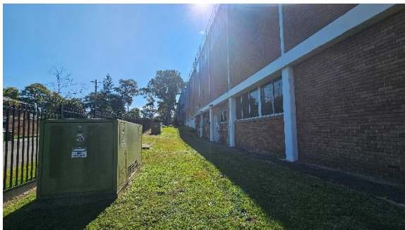
Figure 2.17 Western elevation of 82 Hughes Avenue.
