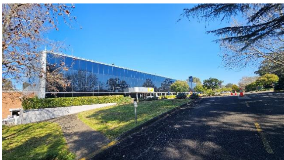
Figure 2.13 Northern elevation of 82 Hughes Avenue.
