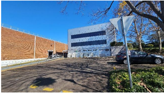
Figure 2.15 Eastern elevation of 82 Hughes Avenue.
