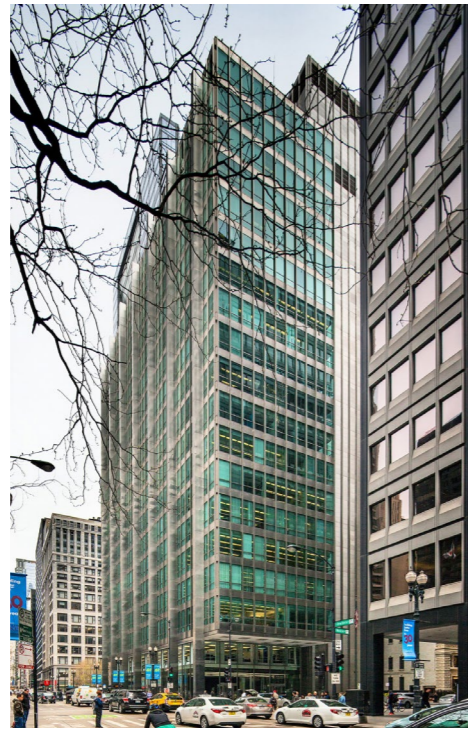
INLAND STEEL / UPGRADE - SOM, 2018
