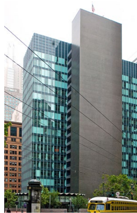
CROWN ZELLERBACH / RETROFIT UPGRADE - SOM, 1990
