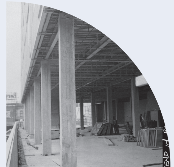
Bates Smart & McCutcheon, MLC Building Construction Progress
