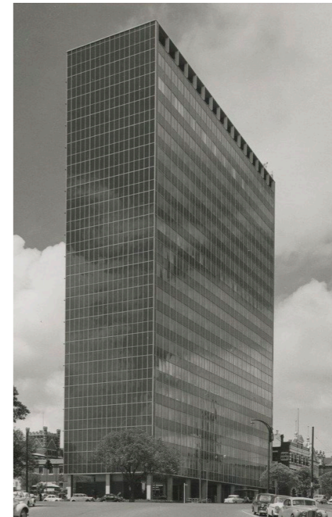
ICI HOUSE, MELBOURNE, 1958 - Bates Smart & McCutcheon
