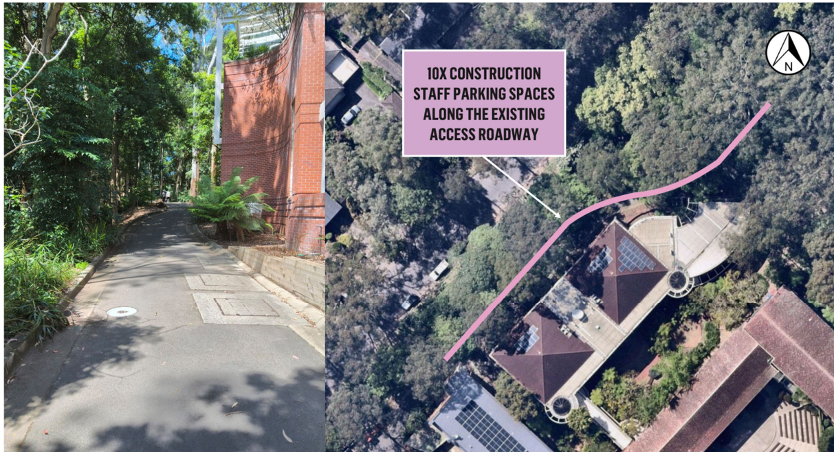
Figure 9 Construction Staff Carpark within the Access Roadway
