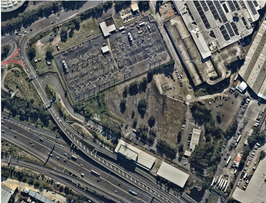
Figure 6 Aerial imagery dated 28 May 2025 depicting the degraded car park surface (Nearmap, 2025)
