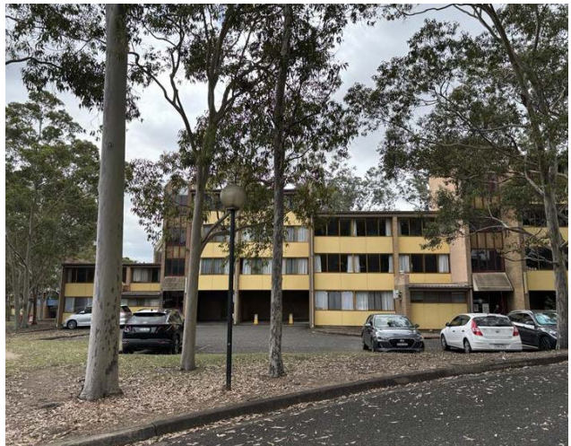
8. Aging residences on Westmead Staff Accommm site.
