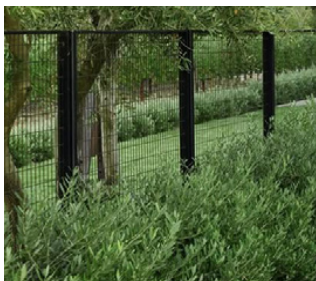
Separation Fencing - 1.8m high palisade
