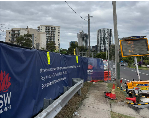
5. Footpath condition near the Alexandra Ave pedestrian crossing.
