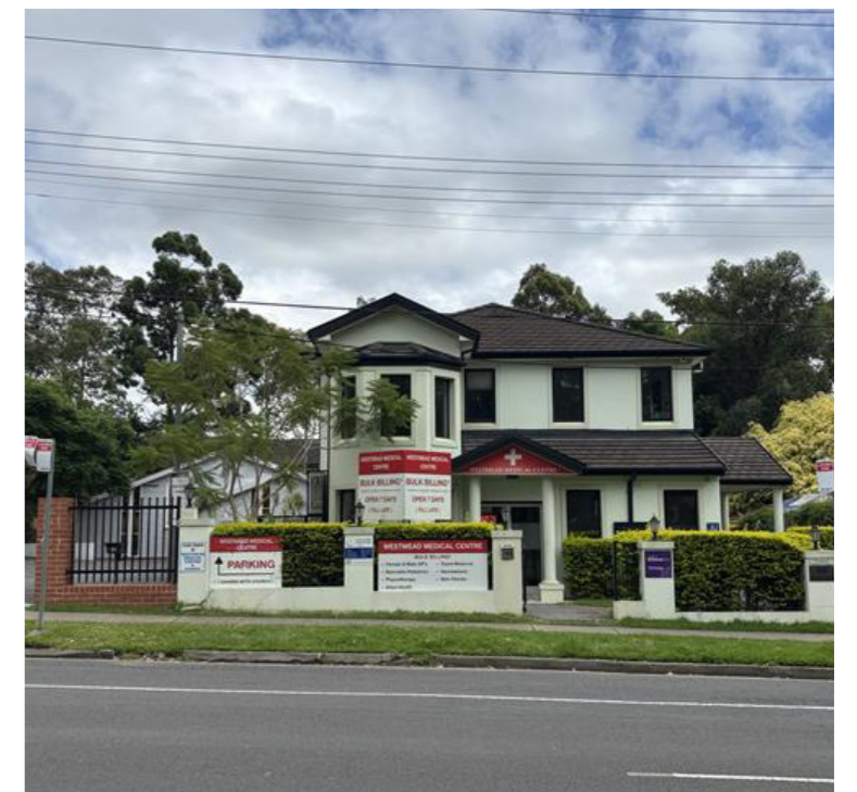
6. View of the 2 storey Westmead Medical Centre on the western side of Bridge Road.
