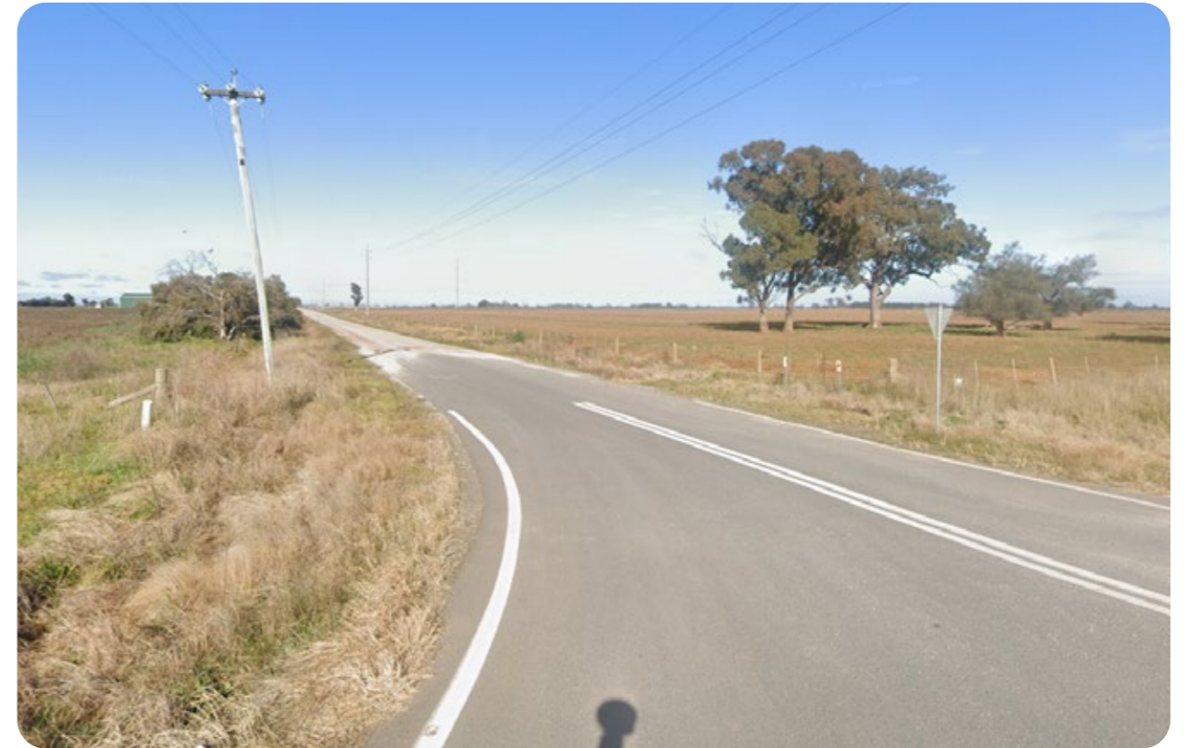
Above: Street view of Canalla Rd showing extent of paved surface from Riverina Hwy.
