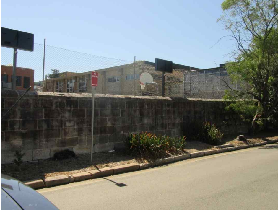
42 Healy Gymnasium and workshop viewed from Luke Street.
