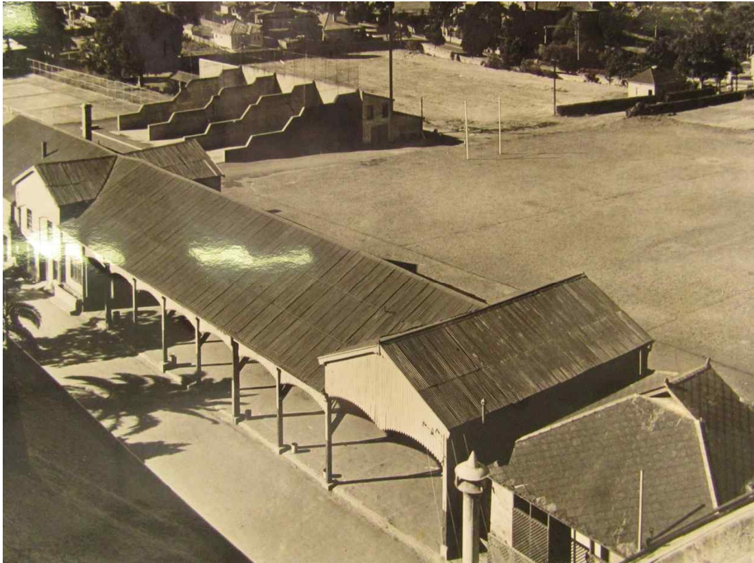
11 Undated photograph of the single storey 1880s building, with the handball courts at upper left. The open nature of the south-eastern section of the College site is apparent. Source: St Joseph's College archives .
