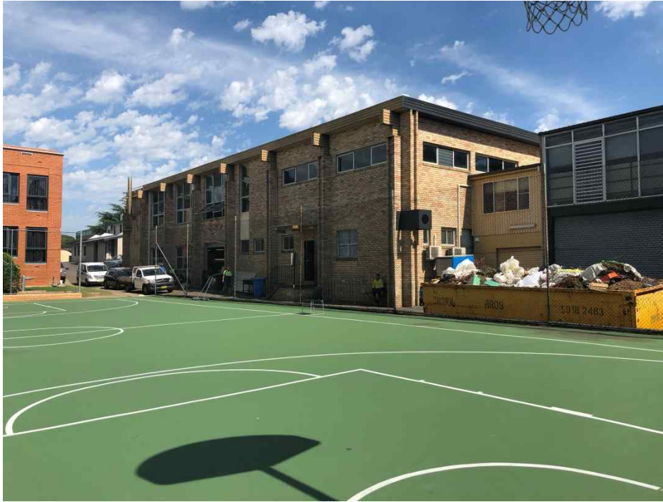
31 Existing Healy Gymnasium viewed from the Sports Courts.
