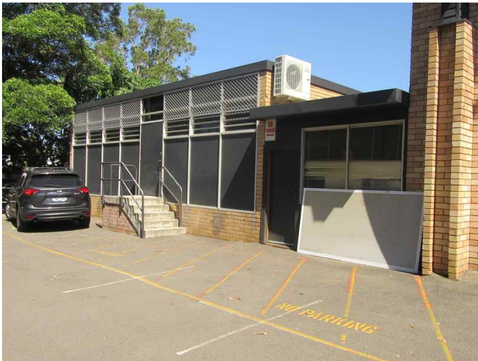
32 Workshop on the eastern side of the Healy Gymnasium.
