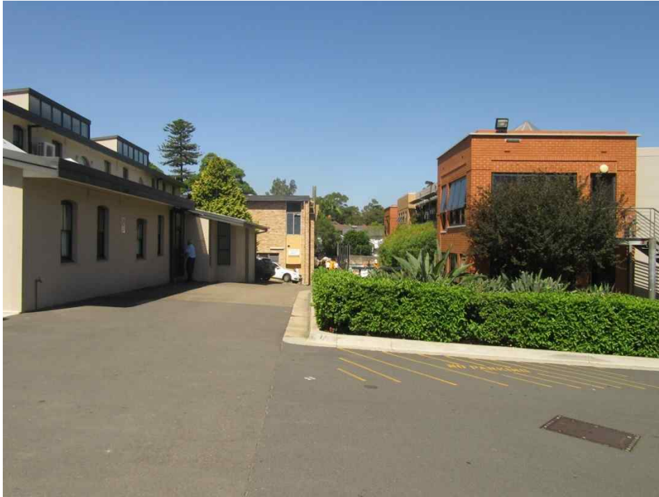
34 Looking towards the Hely Gymnasium from the west. Part of the Year 11 dormitory is visible to the right.
