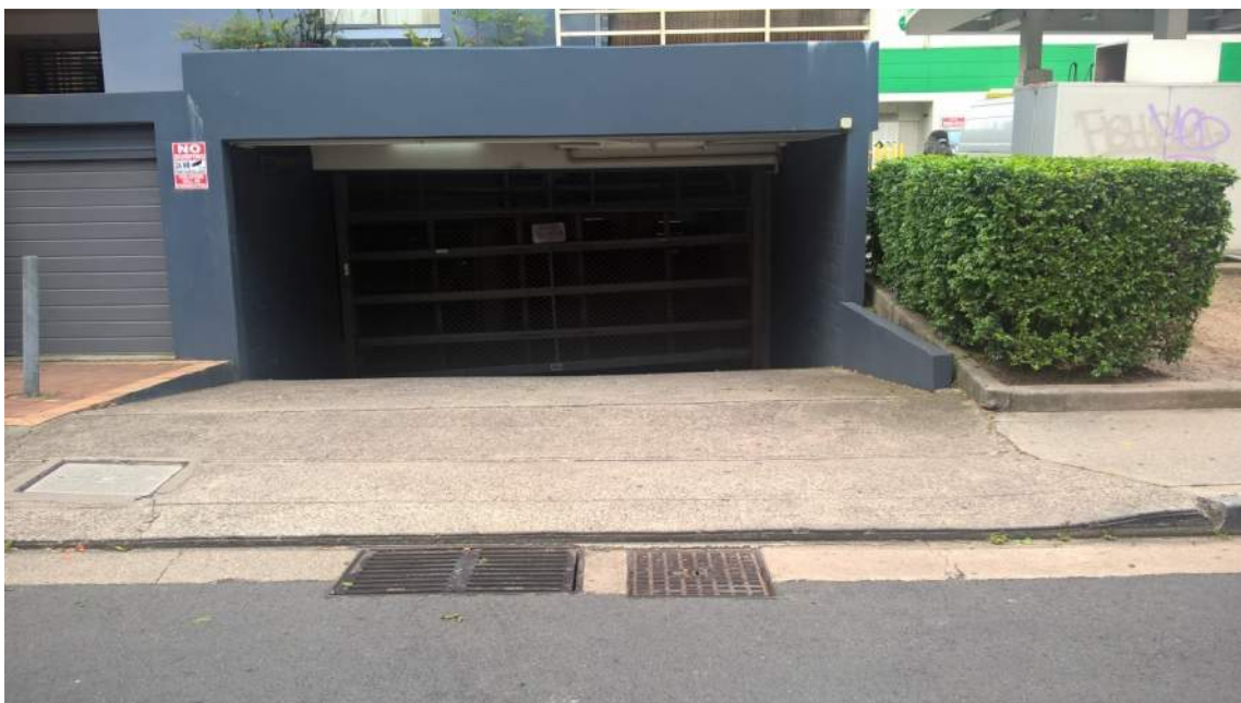
Photo showing existing City of Sydney Council's kerb inlet pit in front of the driveway
