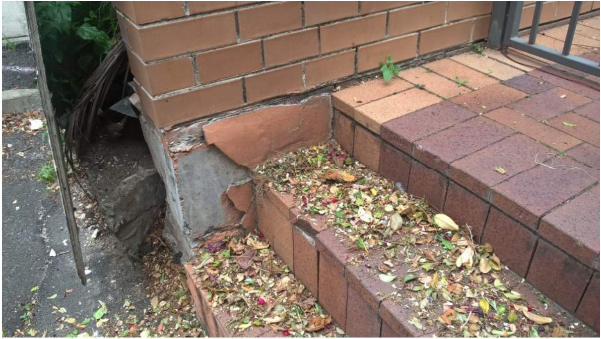
Photo taken from William Lane showing damaged retaining wall.
