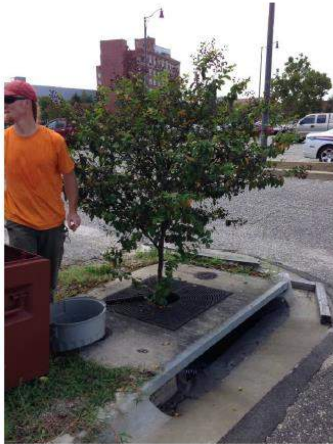
Figure 3. Filterra® at city-owned Amtrak™ parking lot in Fayetteville (Anderson and Smolek, 2015).
