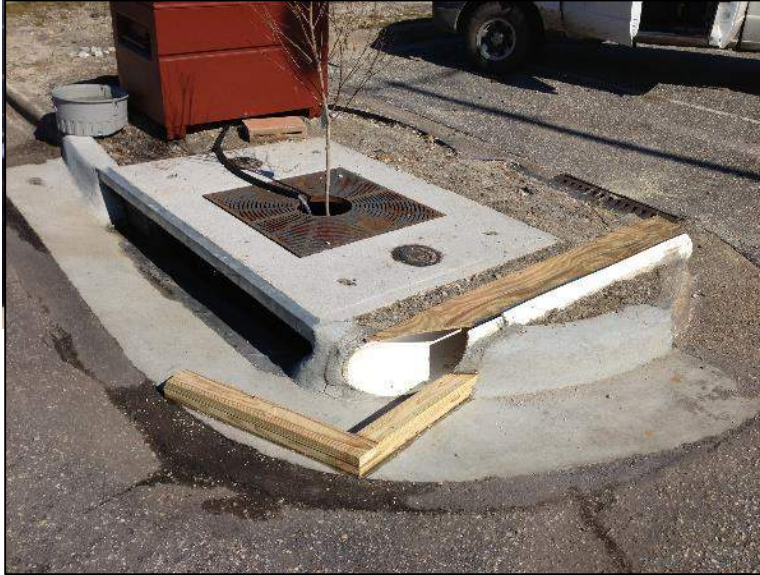
Figure 20. Filterra Site with overflow bypass pipe
