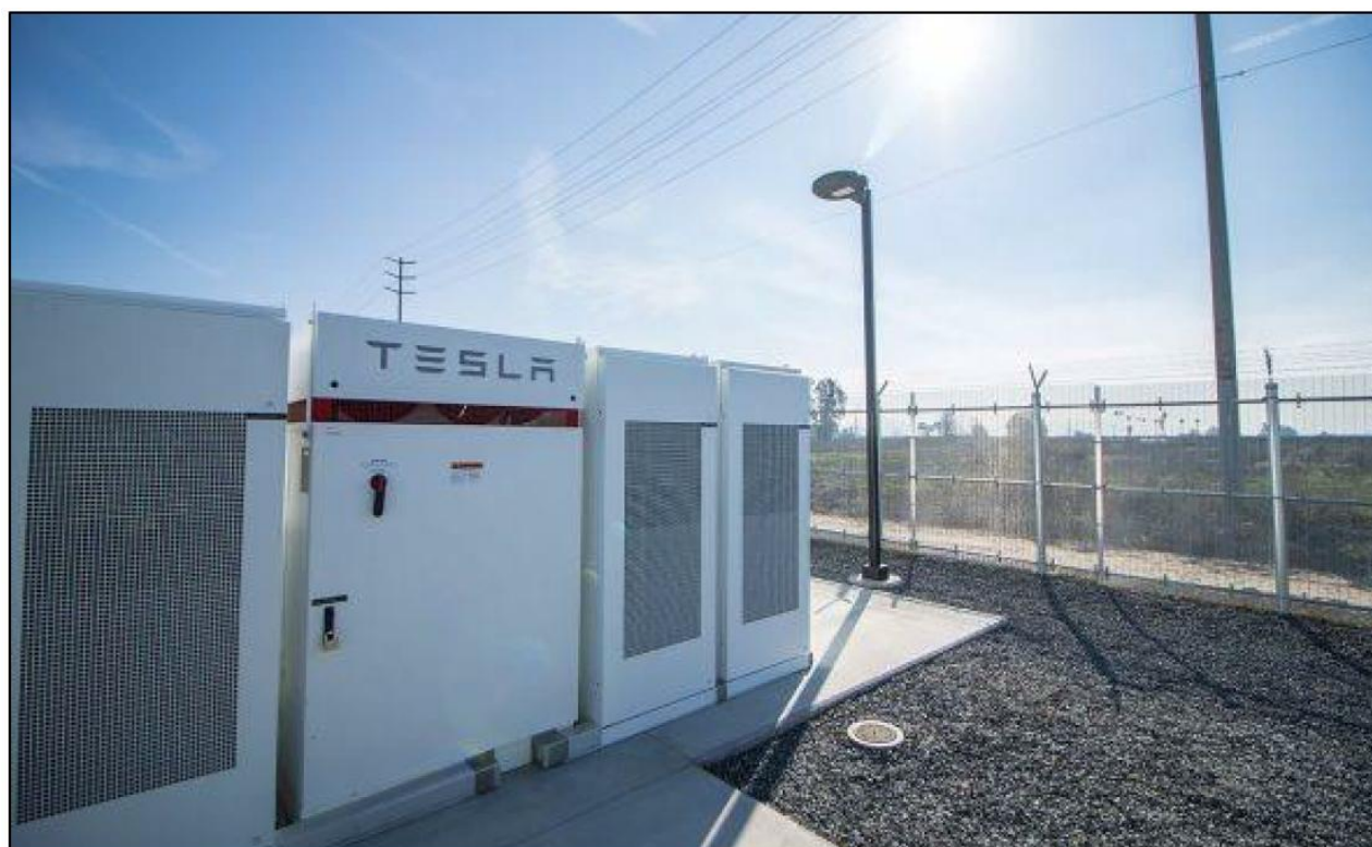
Figure 3-4: Typical BESS
