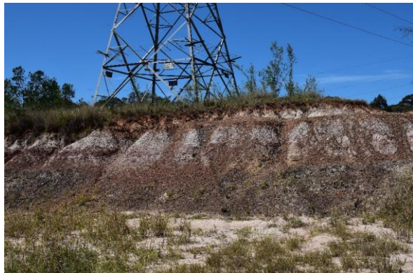
Figure 10: View southeast towards gravelled mound of transmission line tower
