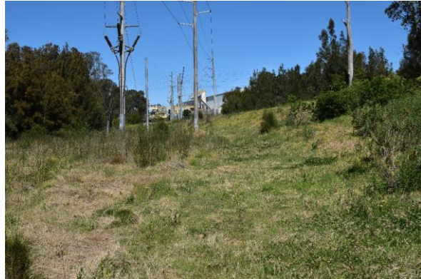
Figure 2: View north of powerline alignment and western elevation
