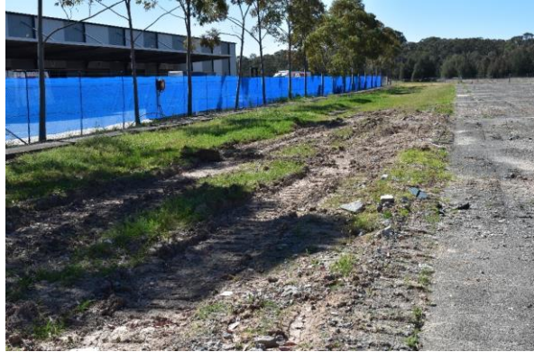
Figure 30: View northeast of fill and lack of soil horizon
