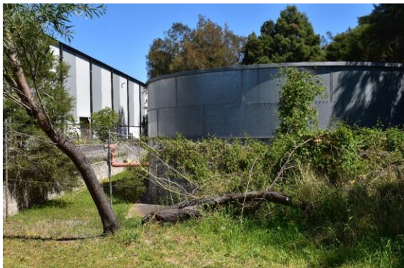
Figure 39: view of water tank at north of property
