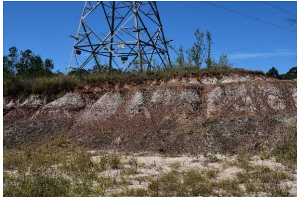
Figure 52: View southeast towards gravelled mound of transmission line tower
