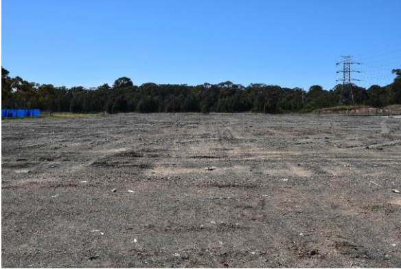
Figure 29: View east of fill after removal of central warehouse
