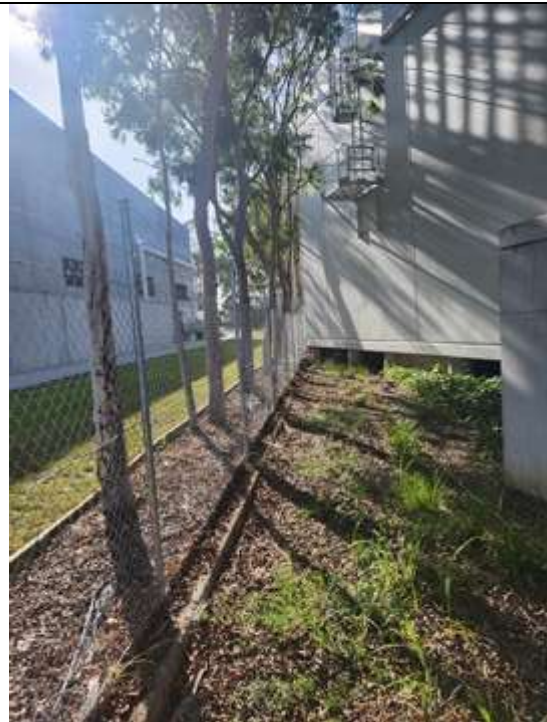
Figure 5 - Photo showing the completed works at 5 Kiora Cres, Yennora, NSW 2161. Image was taken on the 8 March 2024.
