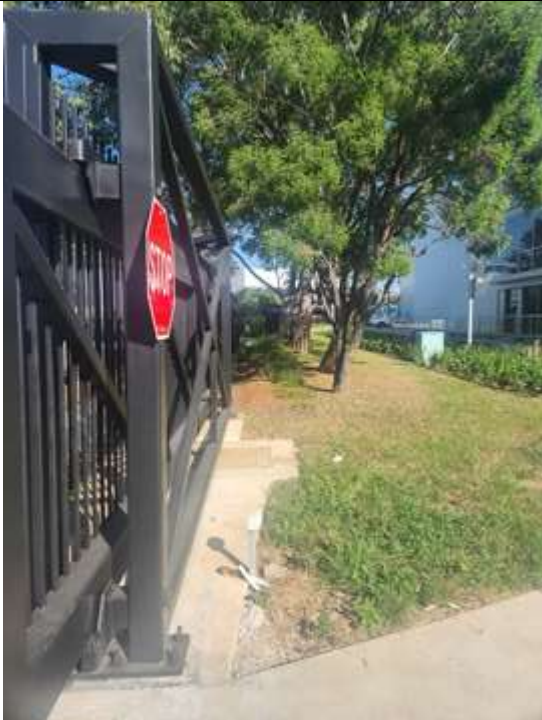
Figure 12 - Photo showing completed works for the front of the sliding gate at 5 Kiora Cres, Yennora, NSW 2161. Image was taken on the 8 March 2024.
