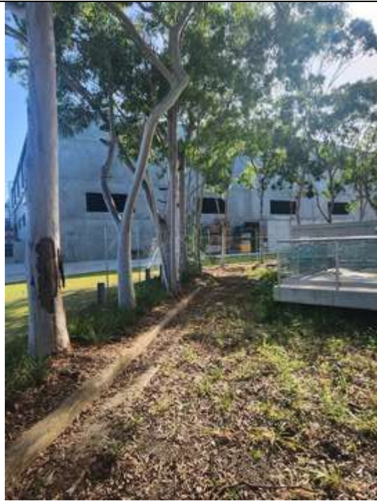
Figure 6 - Photo showing the works at 5 Kiara Cres, Yennora, NSW 2161. Image was taken on the 8 March 2024.
