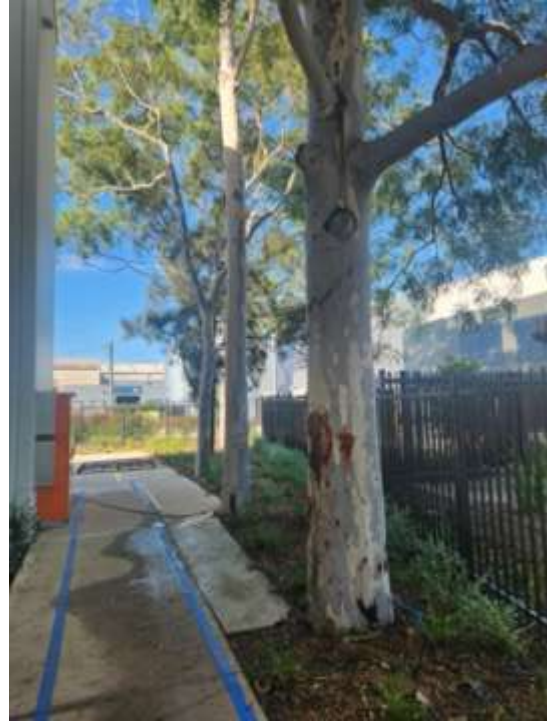
Figure 11 - Photo showing completed works occurred at 5 Kiora Cres, Yennora, NSW 2161. Image was taken on the 8 March 2024.
