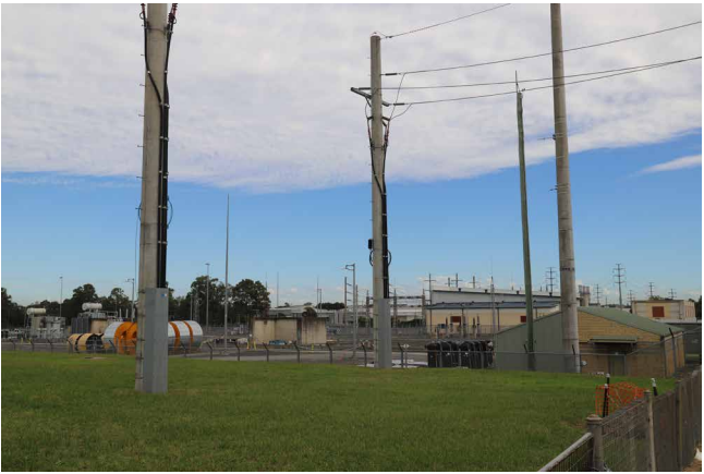
Photo 7. View south-west from 120 McCredie Road.
