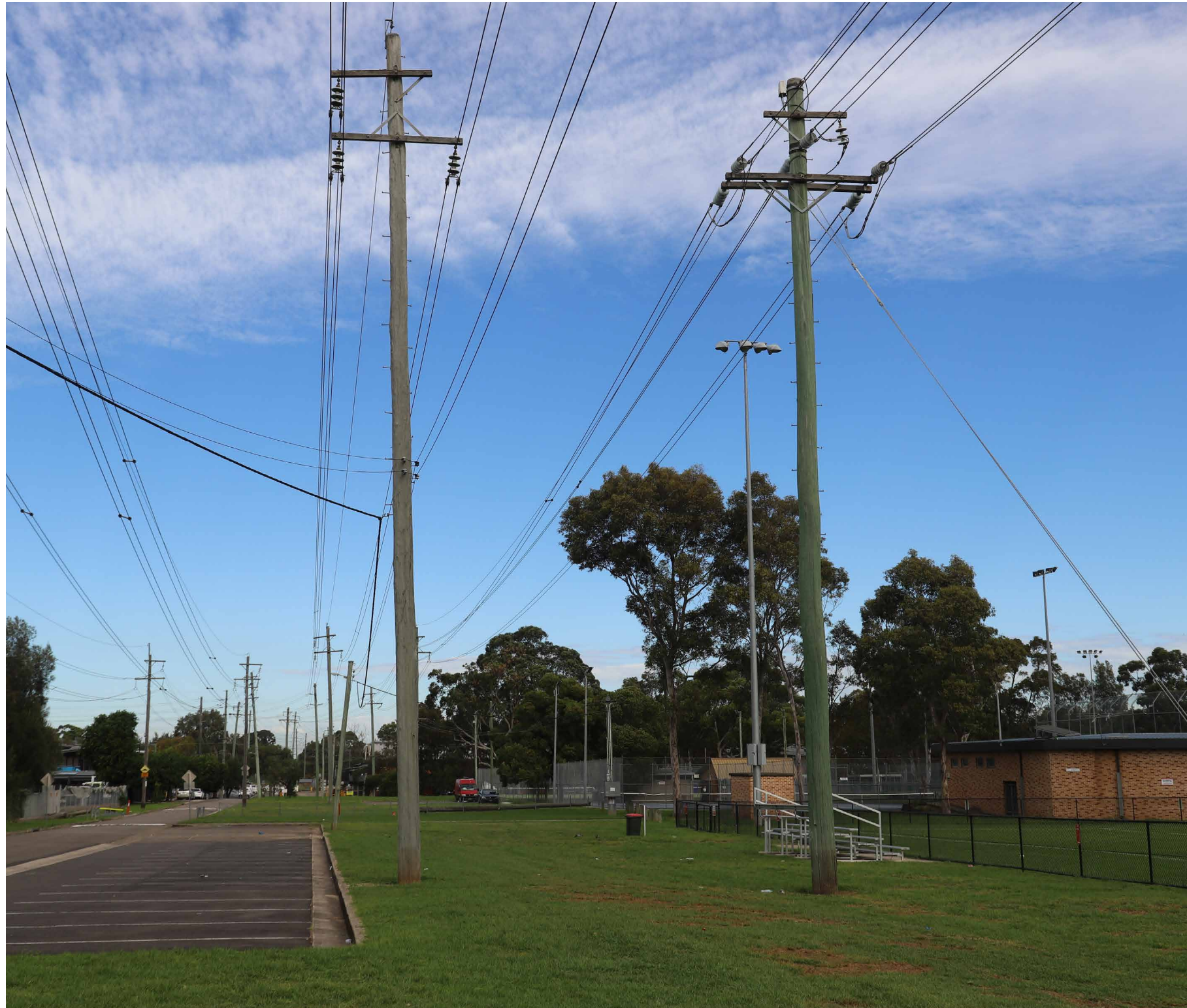
Photo 24. Eastern parking area of Guildford West Sportsground.
