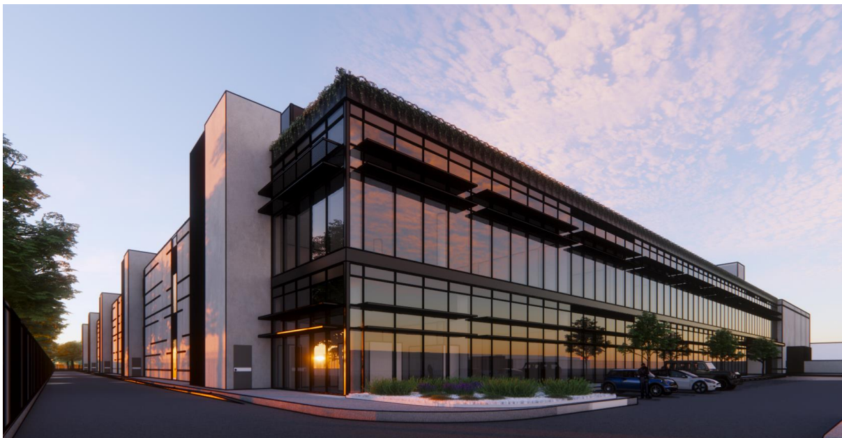
Figure 6 Office facade - July 2025
