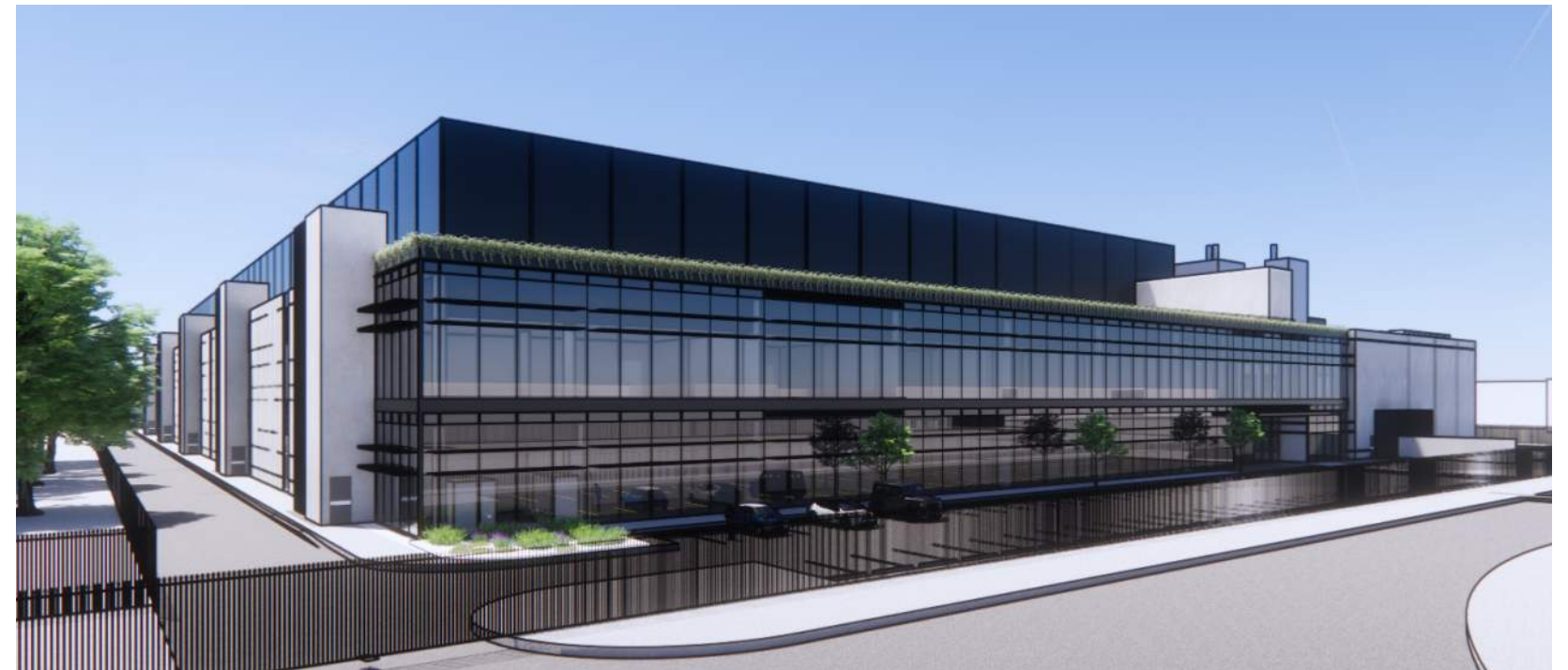
View of the front facade
