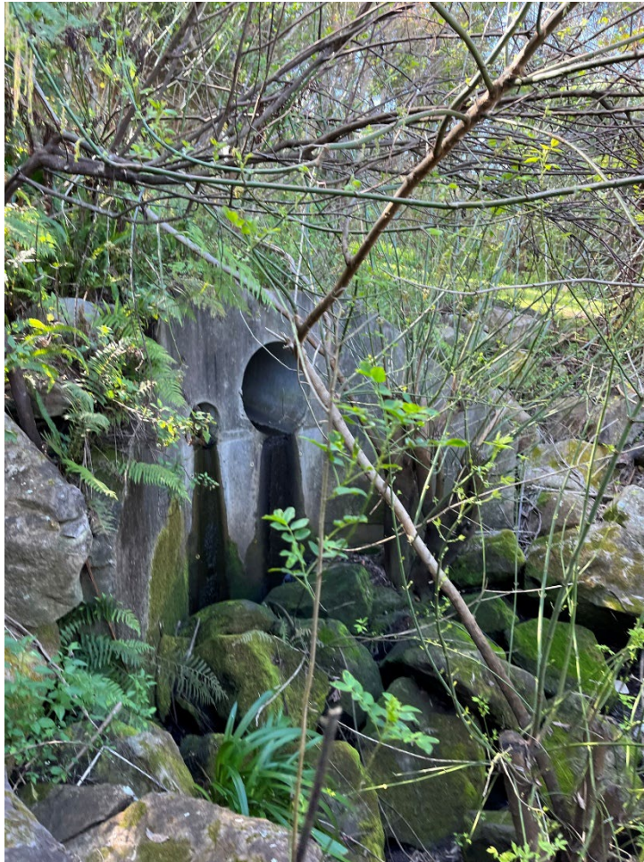
Plate 1. Small culvert drain that occurs within the Subject Property
