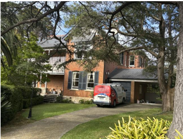
Figure 64 1 Valley Road, Lindfield
