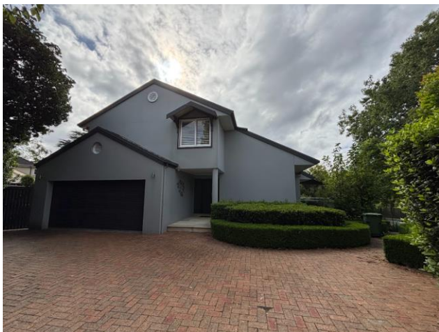
Figure 25 Primary façade of 63 Trafalgar Avenue accessed via a battle-axe driveway
