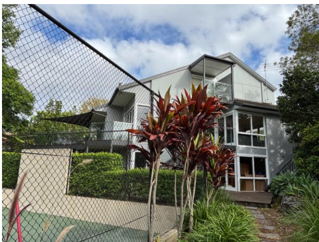
Figure 27 Rear façade of three-storey 63 Trafalgar Avenue
