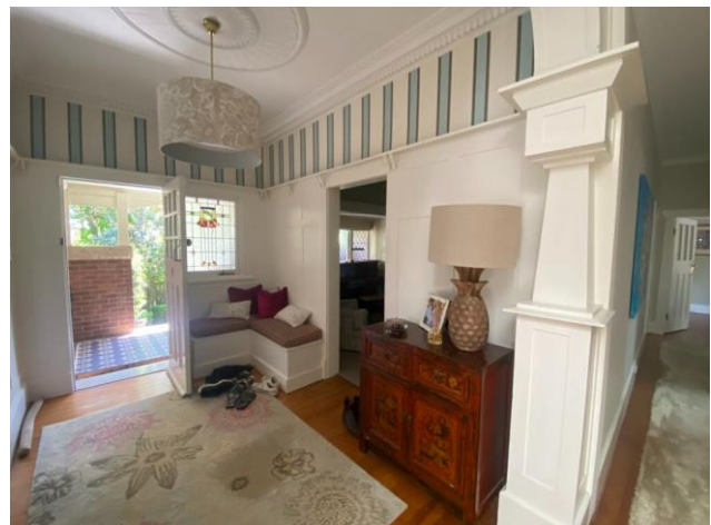
Figure 18 Original front entryway featuring original cornices, ornate ceiling rose, sidelight lead light glazing and ornate portal archway.
