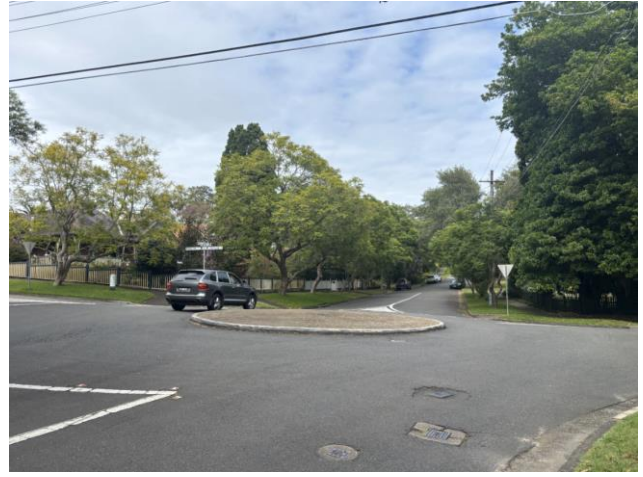
Figure 4 Intersection of Trafalgar Avenue and Middle Harbour Road, looking south Source: Urbis, 2025
