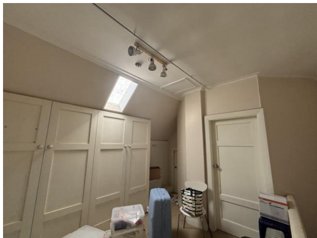
Figure 44 Contemporary undocumented upstairs addition of a bathroom and bedrooms
