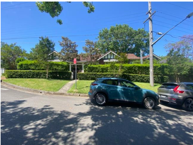
Figure 15 Front façade of subject dwelling from across Trafalgar Avenue.
