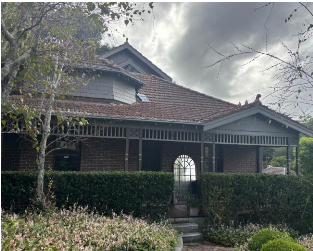
Figure 5 Primary façade with extensive contemporary roof insertions
