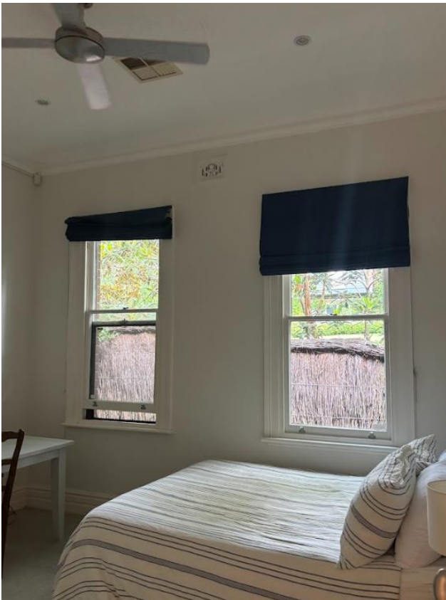
Figure 11 Original bedroom 3 with two original single hung sash windows, skirting boards and air vents
