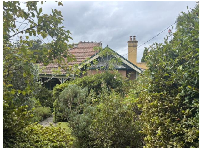
Figure 65 3 Valley Road, Lindfield
