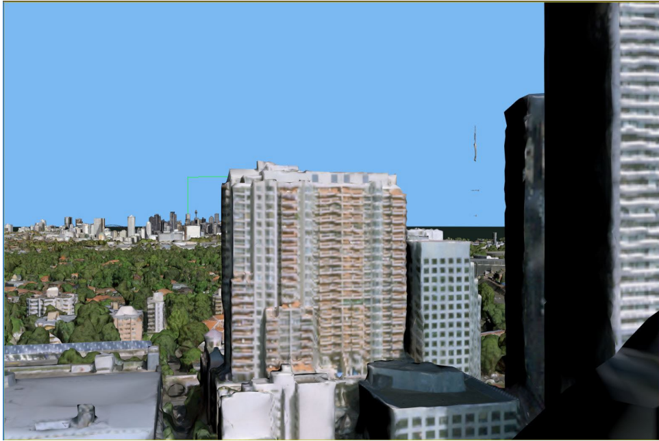
Figure 52 Regency Towers (west tower), southern elevation, upper levels, looking south, existing view
