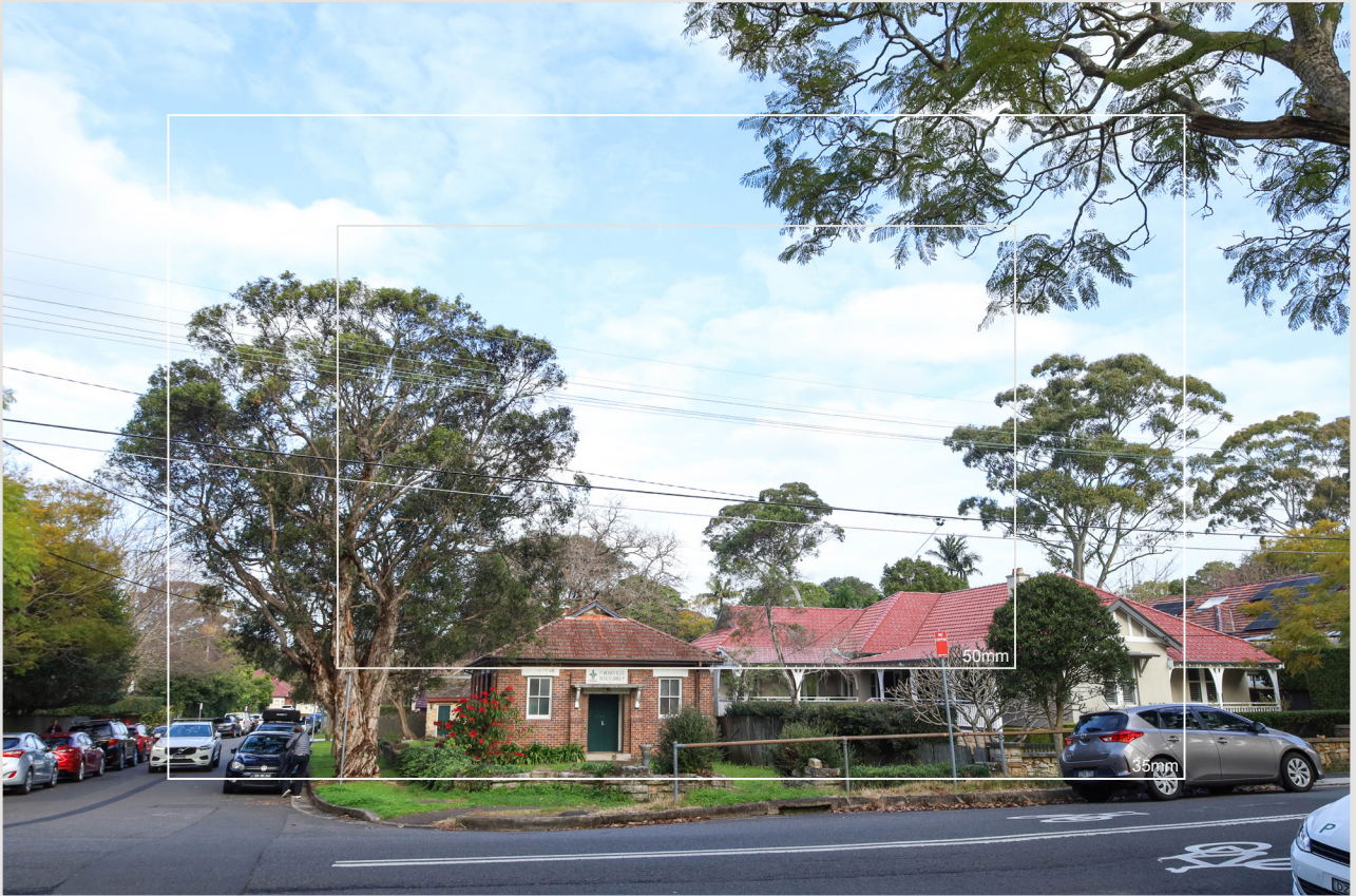
Existing site photo: Corner of Lord Street and Martin Lane
