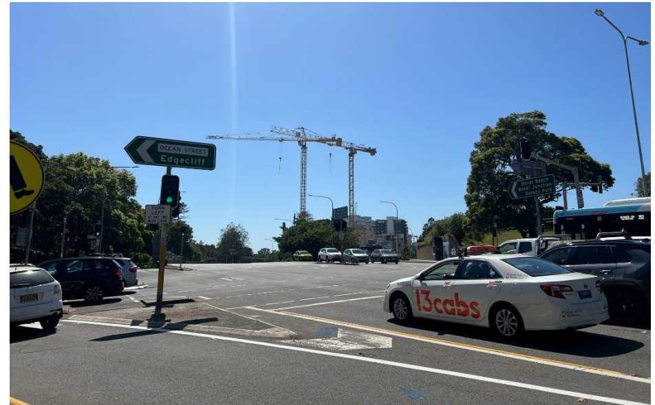
Figure 12: Looking east towards the site from cnr Ocean Rd/ Oxford St (Source: Keylan)
