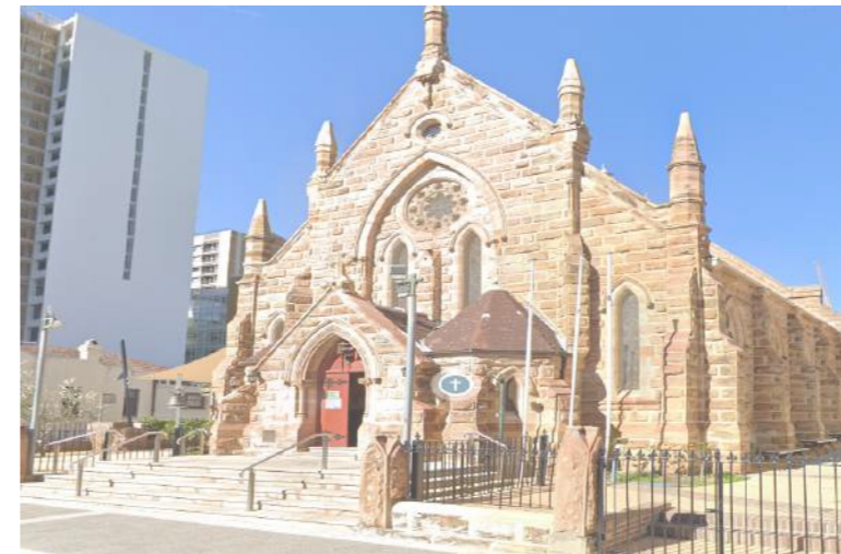
Adjacent heritage church
