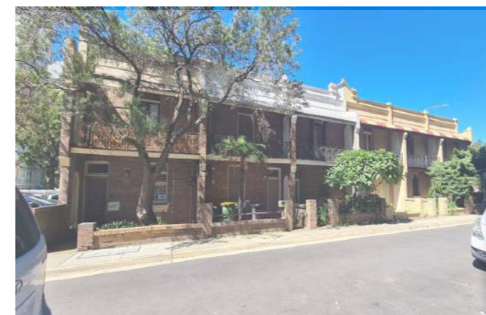
Item 3 - Attached dwellings no. 12-22 Burleigh St
