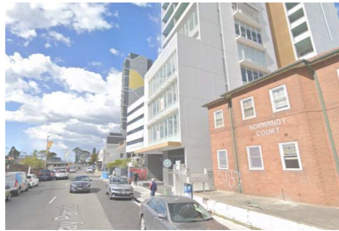
awning at 10-16 Railway Pde
