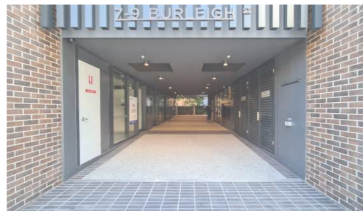
Through-site link of no. 7-9 Burleigh St to Burwood Rd
