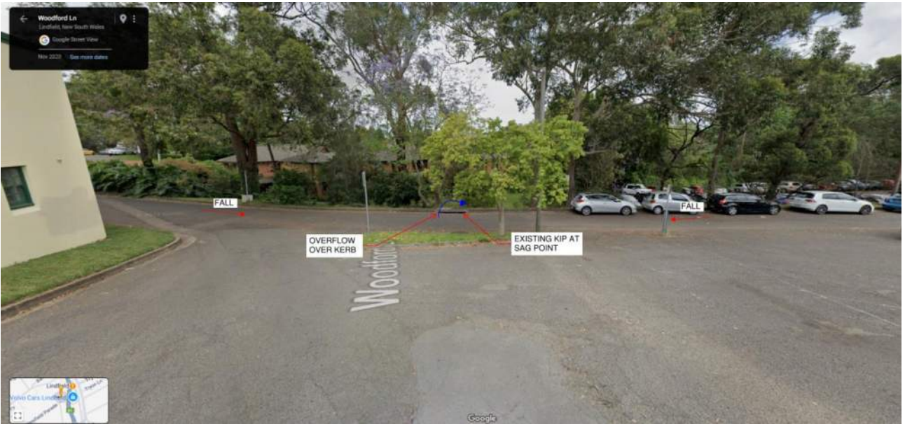
Figure 5 Sag Point Kerb Inlet Pit at Upper Carpark
