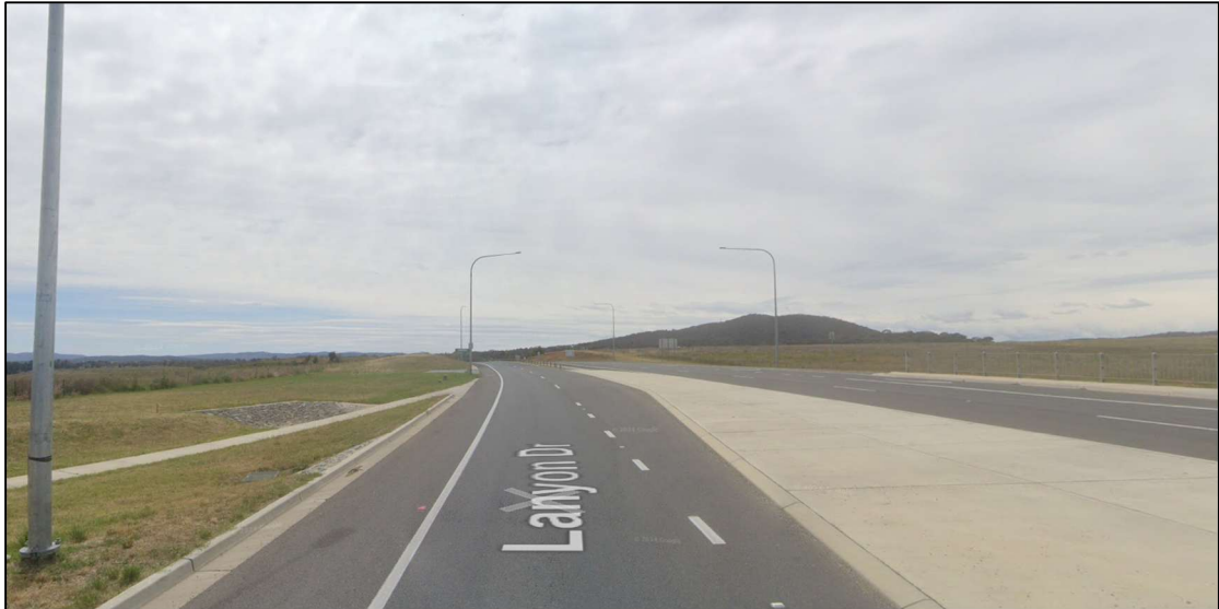
Figure 10 - Lanyon Drive (facing north-east)
