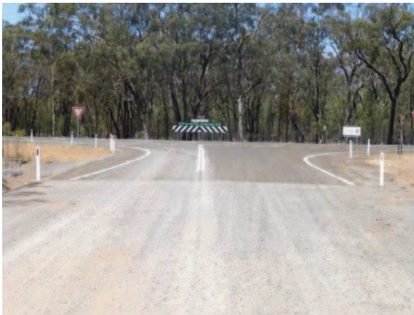
Plate 3-9 Leewood – Old Mill Road looking toward intersection with the Newell Highway
