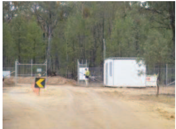
Plate 3-8 Leewood – site entrance looking towards from the site
