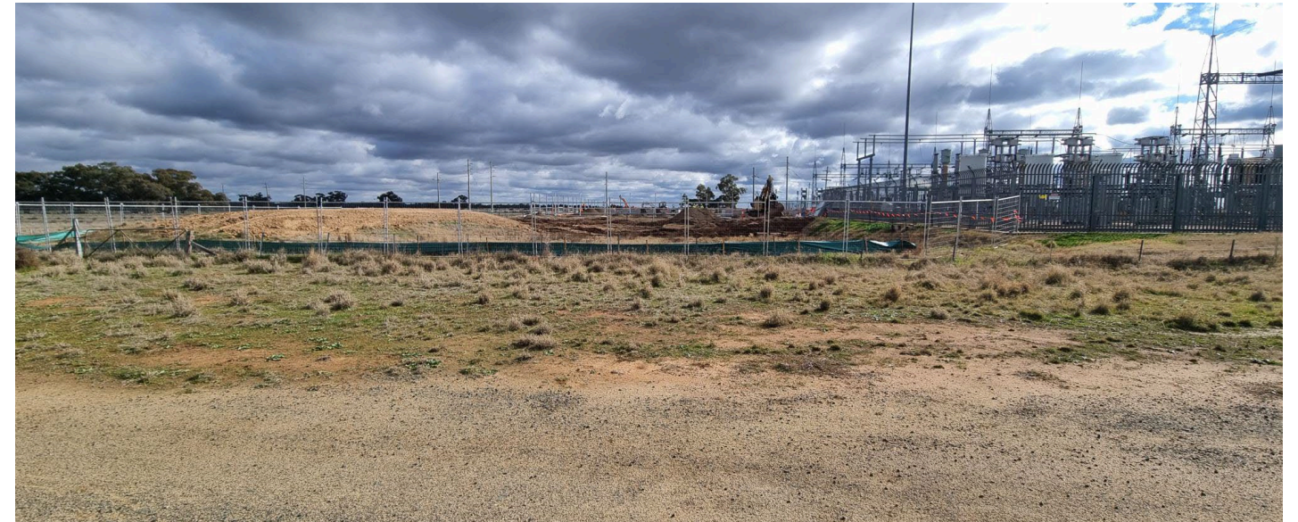
Figure 14-8 Construction works observed within the Deniliquin substation
