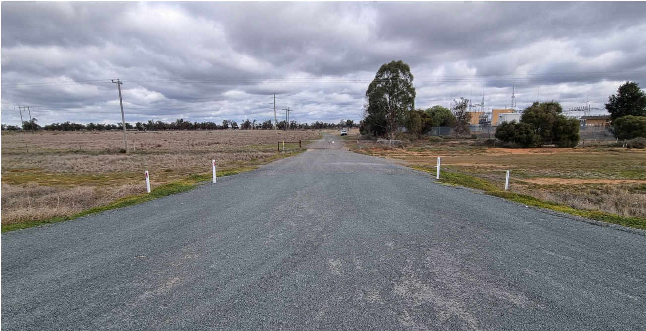
Figure 14-1 Development site access road (view from the Riverina Highway)
