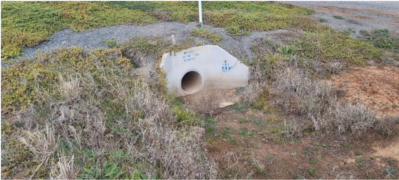
Figure 14-3 Culvert observed intersecting the Development site access road
