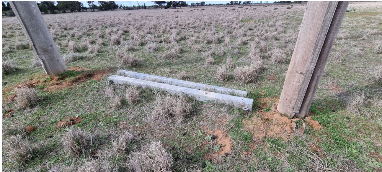
Figure 14-7 Scrap metal observed within proximity to existing powerline infrastructure
