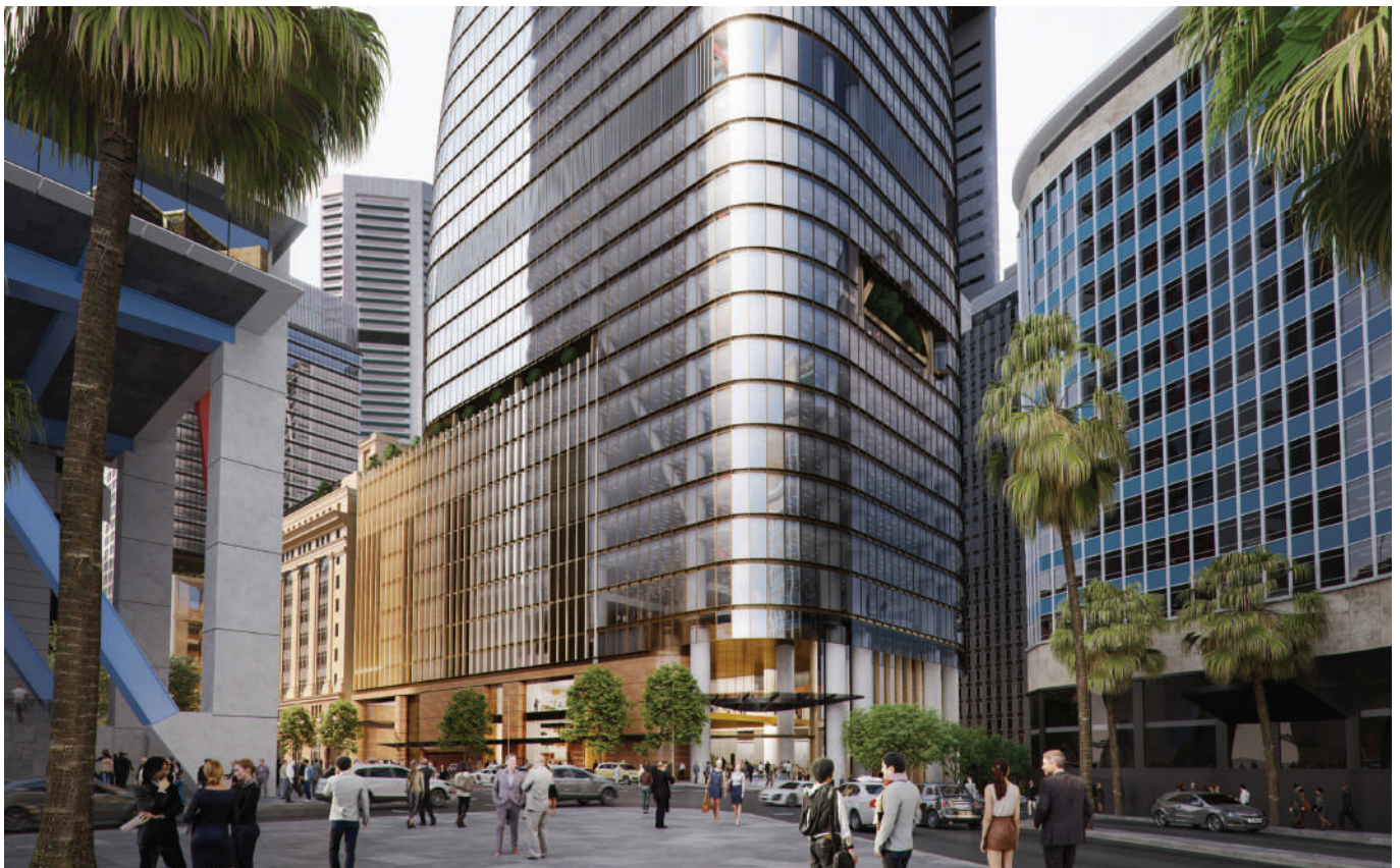
Figure 7. Elizabeth Street and Hunter Street corner Metro entrance public domain interface
