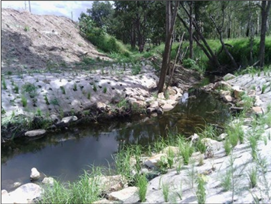
Plate 2 - Bundamba Creek Regeneration works (Australian Wetland Consulting, 2018)
