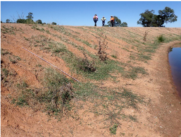
Figure 38 – Example of exposure in SU3 around the dam, facing W.
