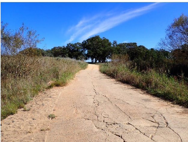
Figure 72 – Concrete causeway over Slapdash Creek; aspect west.
