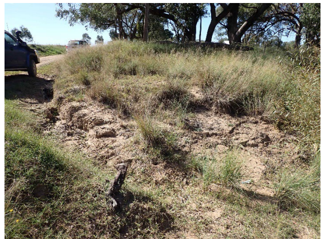
Figure 71 – Modified creek bank at creek crossing on Jacksons Lane; possibly eroded subsoil; aspect north-east.
