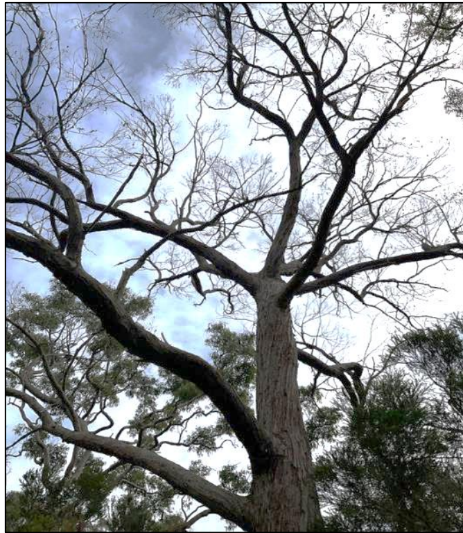
Plate 3 Above: Tree 386 – Eucalyptus globoidea showing poor health. This tree has a SULE of <5 years and should be removed.
