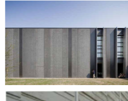
PRECAST CONCRETE WALL
