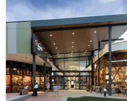
METAL FRAMED GLAZING
