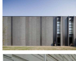
PRECAST CONCRETE WALL
