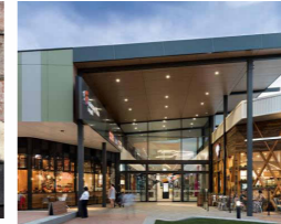
METAL FRAMED GLAZING
