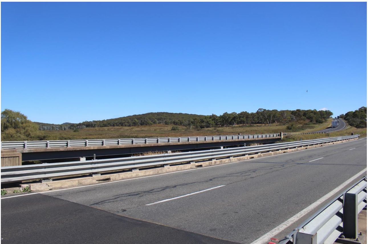
Figure D.4 Rehabilitated view
