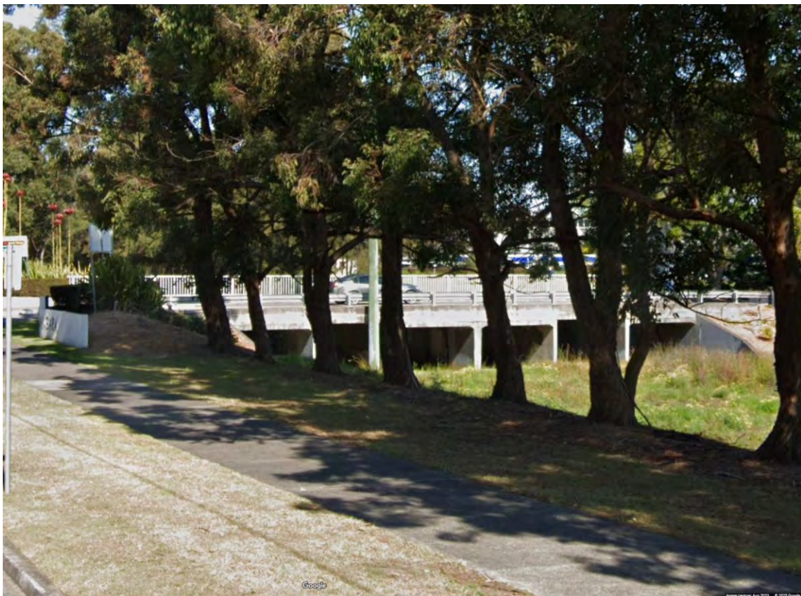
Figure 6 Moss Drain culverts looking upstream (Source: Google street view)
