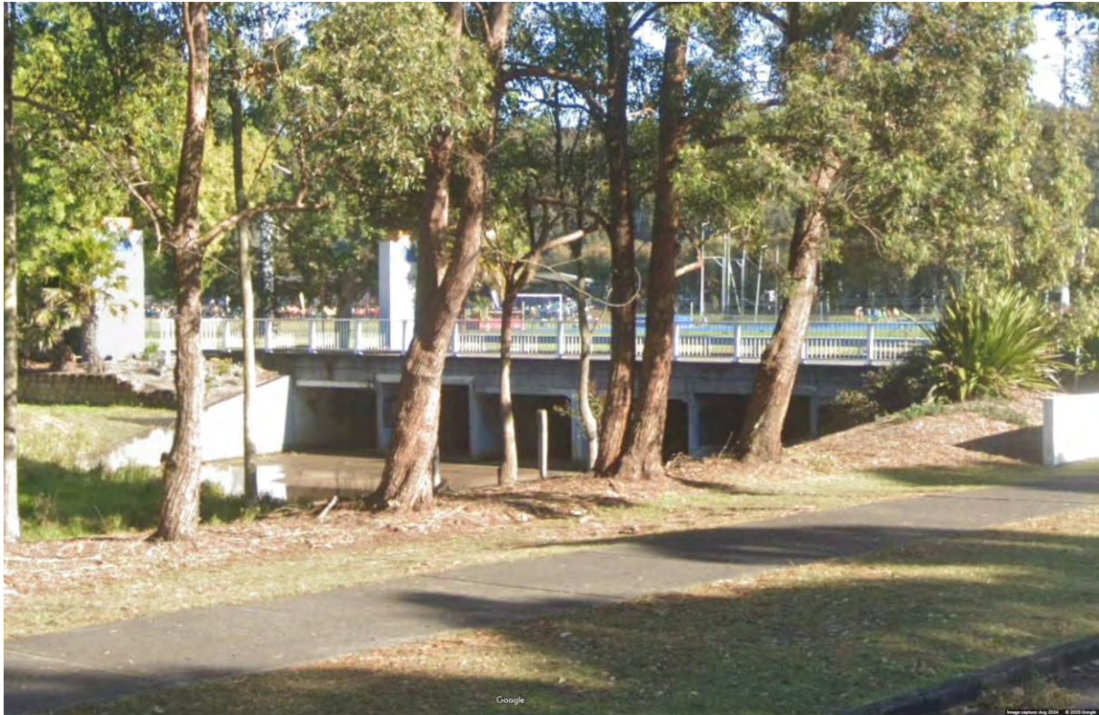
Figure 5 Moss Drain culverts looking downstream (Source: Google street view)
