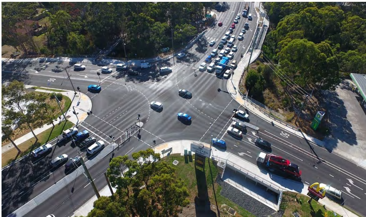
Figure 4 Mingara Drive culverts (source: https://cmc.net.au/projects/wyong-road-upgrade/ )
