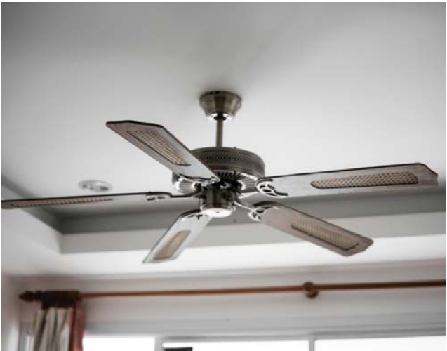
Provide ceiling fans to enhance air circulation
