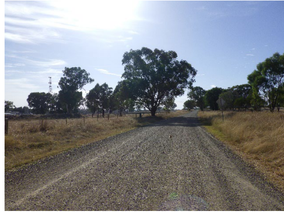
Figure 5 – Boiling Down Road (view east)
