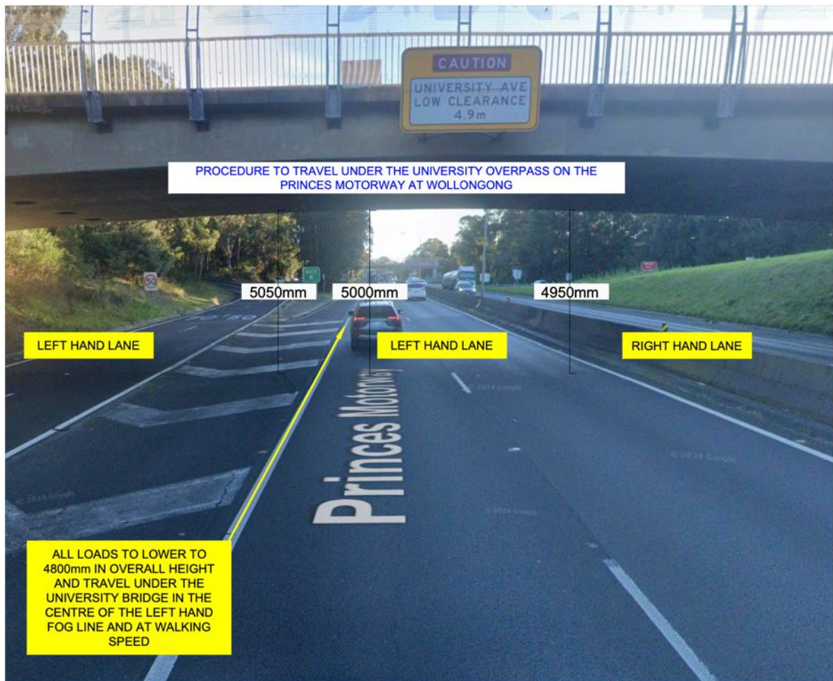
Figure 10 - University Overbridge on the Princes Motorway for loads under 4.8 metres in overall height
