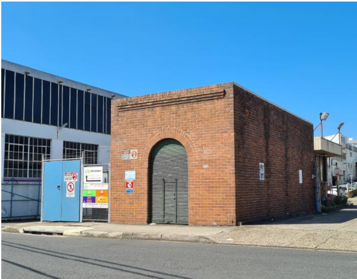
Figure 1: Existing Ausgrid ground substation S.370 William Street (March 2024)
