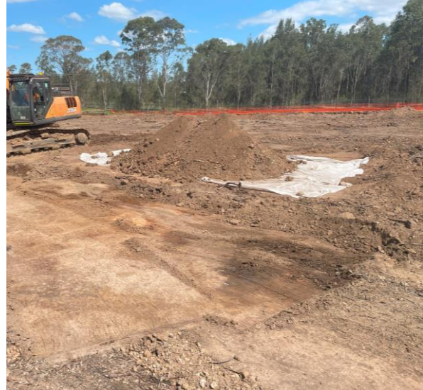
Photo 2: SP24 ground surfaces comprising natural soil following remediation (21 November 2024)
