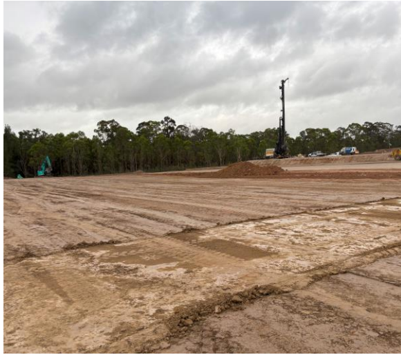
Photo 5: SP24 final inspection following complete removal (31 January 2025)
