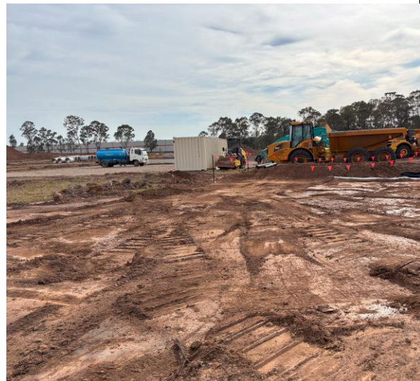
Photo 4: SP24 ground surfaces comprising natural soil following additional removal (3 December 2024)
