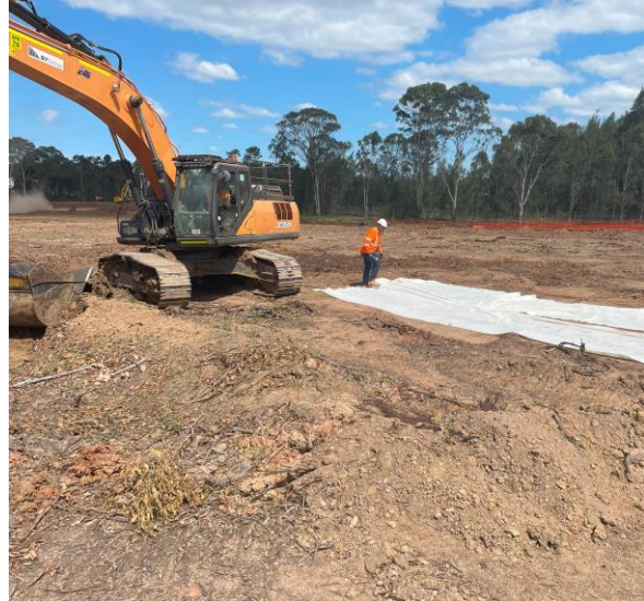
Photo 1: SP24 removal and placement on geofabric (21 November 2024)
