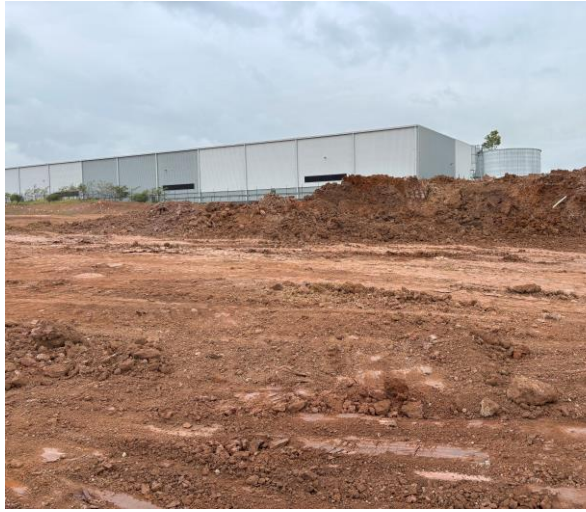
Photo 9: SP25 ground surfaces comprising natural soil following remediation (31 January 2025)
