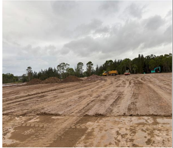
Photo 6: SP24 final inspection following complete removal (31 January 2025)
