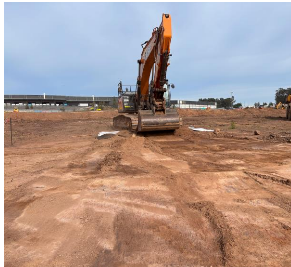
Photo 3: SP24 additional removal and placement on geofabric (3 December 2024)
