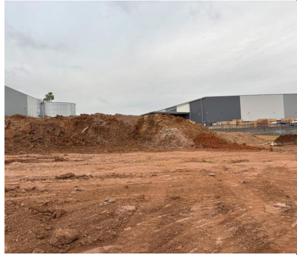
Photo 10: SP25 ground surfaces comprising natural soil following remediation (31 January 2025)
