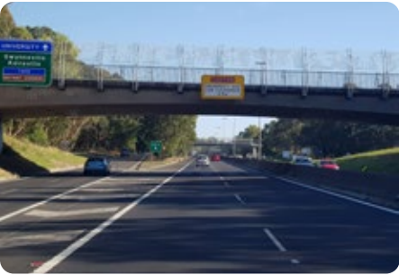
Above: University Avenue overpass of M1 Motorway - 5.2m clearance in left hand lane
