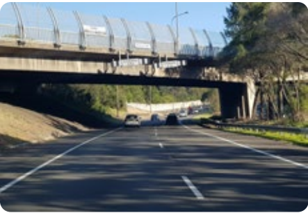
Below: Princes Hwy overpass of M1 Motorway - 5.3m clearance in right hand lane
