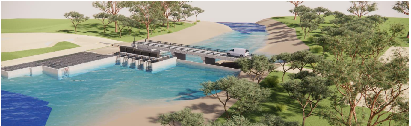
Figure 1.2: Indicative layout of a regulator
