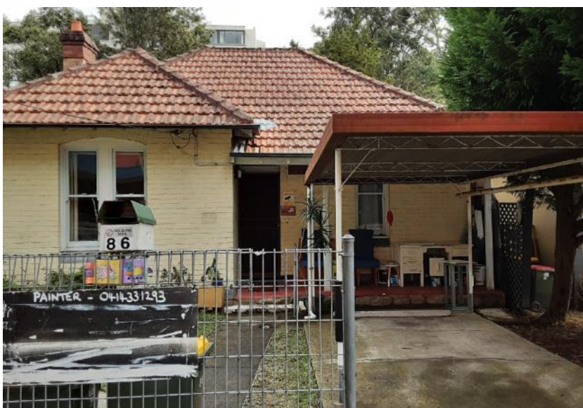
Photo 20 Residential property within Lot 1 DP19887, facing south-east
