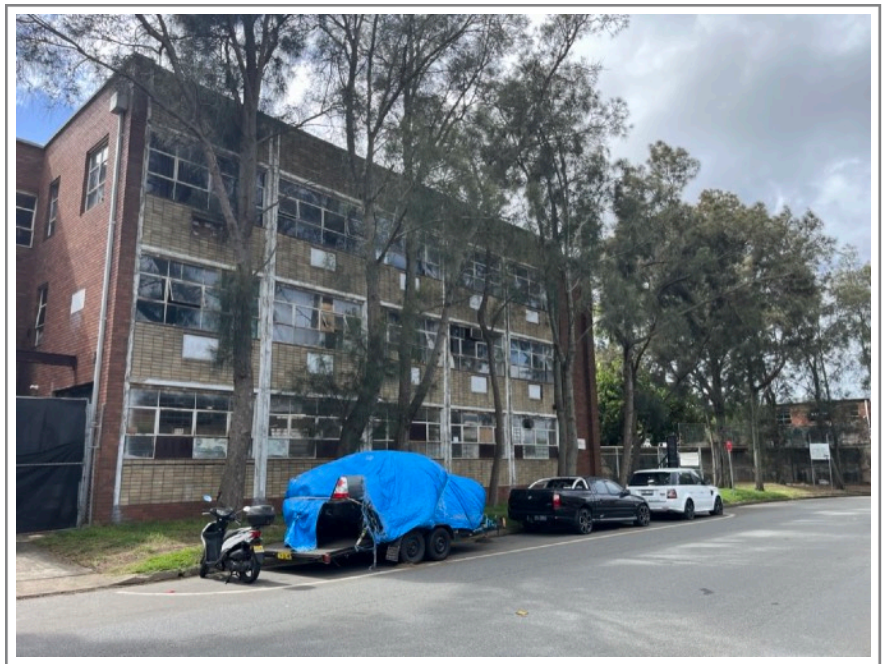
Figure 3 Shows part of the stand required for removal to allow vehicular access.
