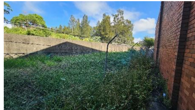
Figure 4. Current site conditions, west of the existing building – set back between existing building and site boundary.
