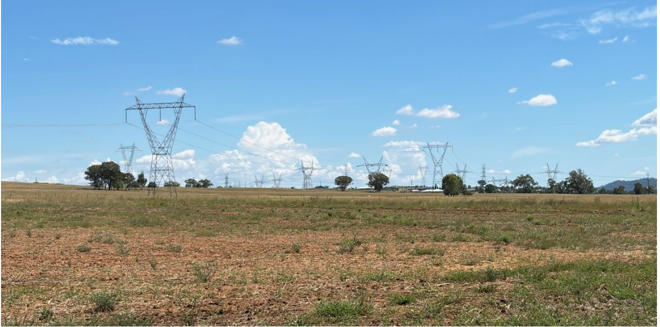
Figure 3-1 Example of steel lattice structure (currently present on the Project Site).
