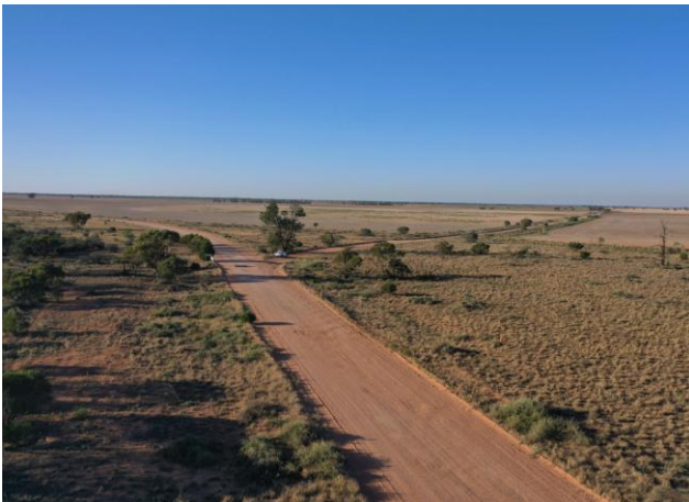
Plate 4-15 View of intersection of the Balranald-Moulamein Road and Arundel Road (Rex J Andrews 2024).
