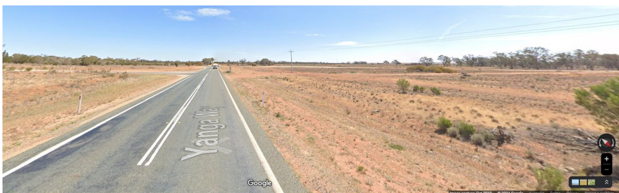
Plate 4-3 View south along Yanga Way towards the intersection with the Balranald-Moulamein Road (from Google Earth Street view).
