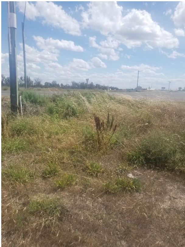
Plate 4-9 View of the intersection of Murray Valley Highway and Sturt Highway, Euston (NGH ecology team photo). Note services.
