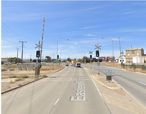
Figure 34: Rail crossing on Eastern Parade at Port Adelaide
