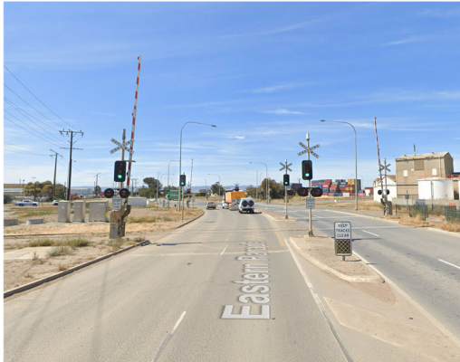
Figure 31: Eastern Parade rail crossing
