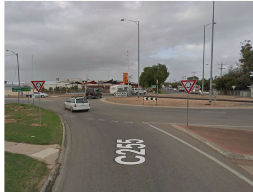
Figure 35: Rail crossing on Benetook Avenue at Mildura
