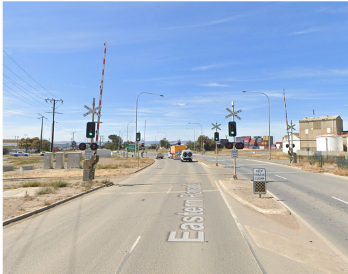
Figure 69: Eastern Parade rail crossing
