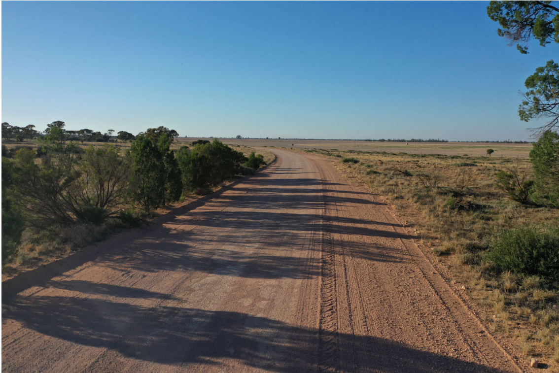
Figure 28 - Typical section of road along Balranald Road, NSW.
